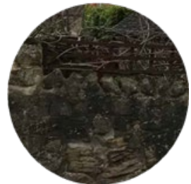
Stone boundary wall
