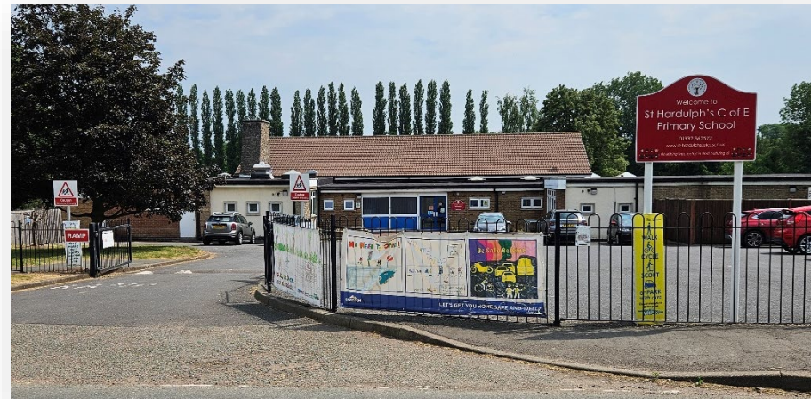
Figure 8: St Hardulph's Church of England Primary School
