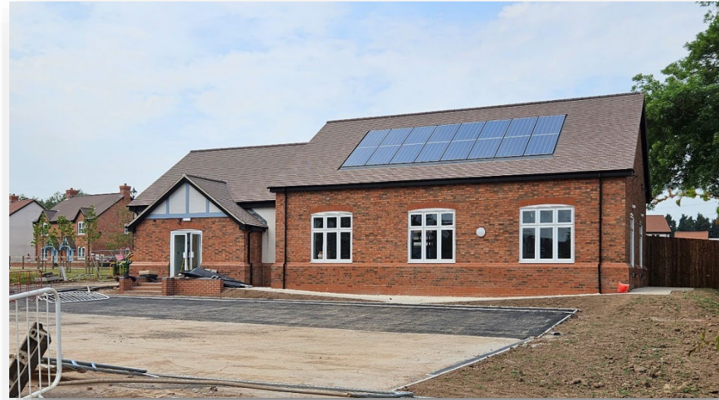
Figure 11: Breedon Village Hall nearing completion
