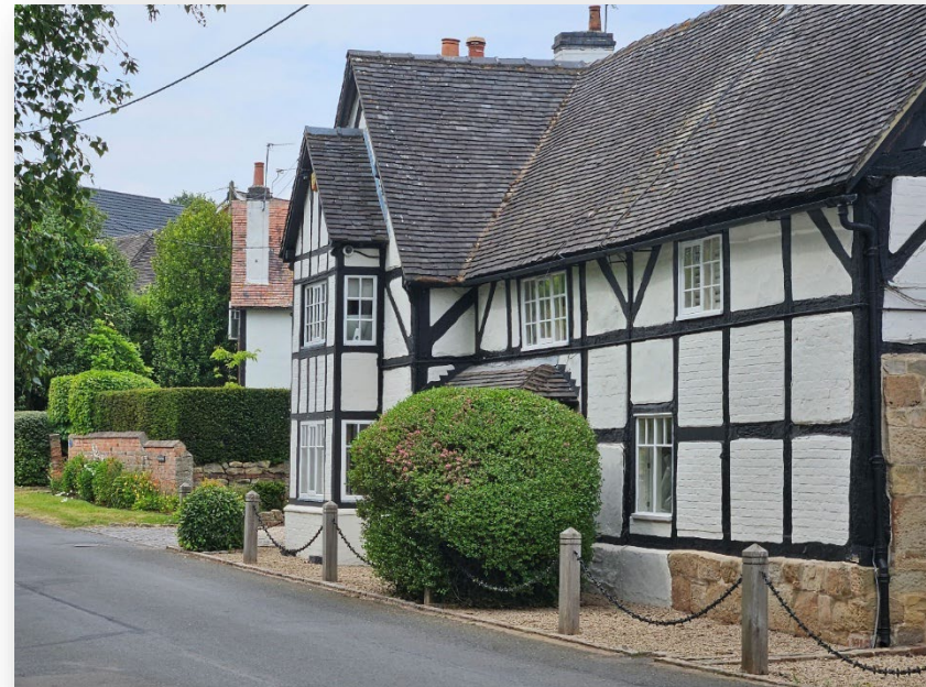
Figure 13: Brook House, Wilson
