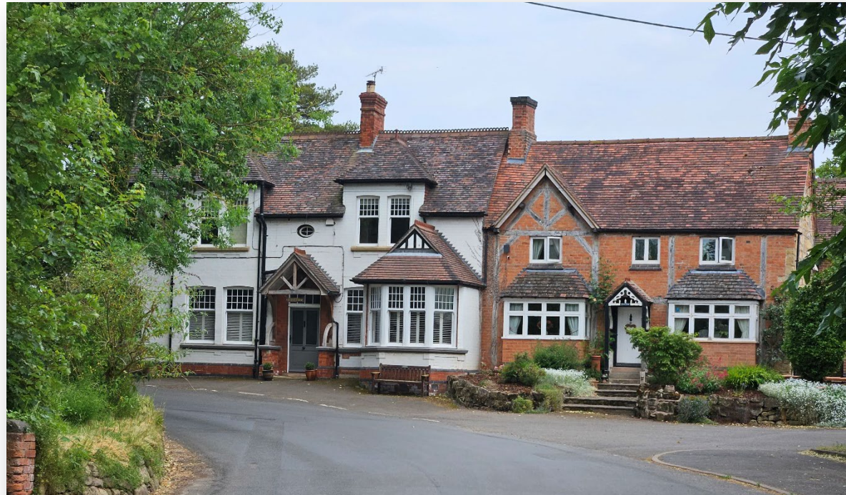
Figure 17: Wilson Conservation Area
