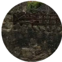
Stone boundary wall
