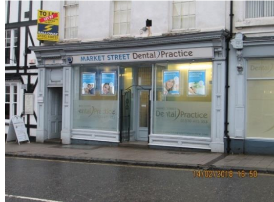
Market Street, Ashby de la Zouch Shop front installed after c.1880
