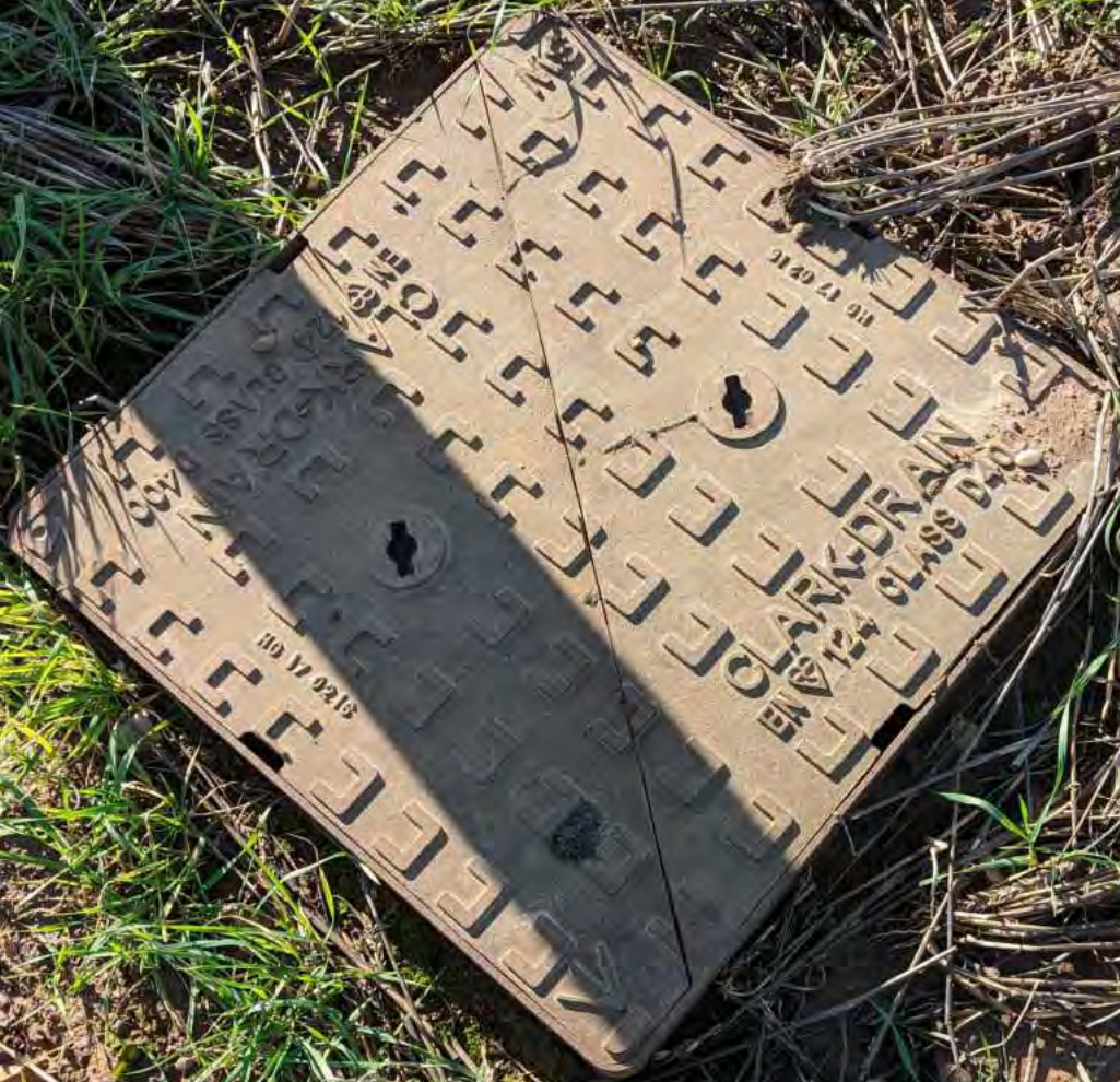
Northern highway drain manhole
