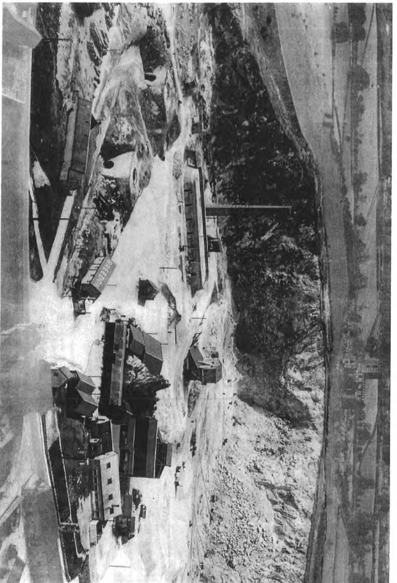
In the centre left of the picture is the "Sercombess" lime kiln which was able to run continuously. In front of it and to the left are the two old round "Hoffman" kilns. The round kilns were changed from the top, with limestone and coal. Only when the fire had gone out and the kiln cooled could the contents be emptied into the waiting tubs. In right centre is the pinnacle with garages grouped around it. 1946
