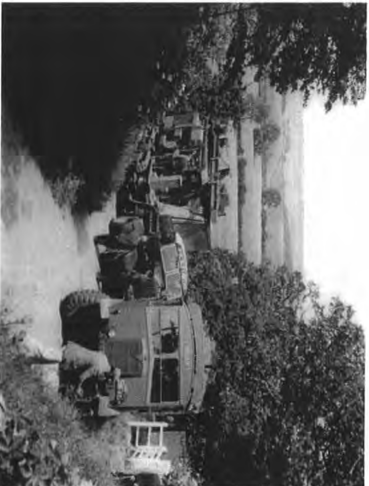
A Ruston Bucyrus RB27 well drill (also known as a bonging iron) was used to make a hole to half the depth of the face for the explosive charge. This method speeded up rock blasting significantly. 1952.
