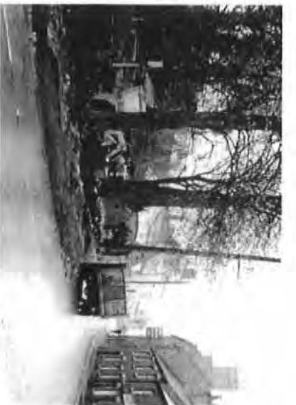
The Hall garden wall at the edge of the road is being demolished and rebuilt ten metres back from the roadside to improve visibility for traffic on the blind corner and to allow a footpath to be created. October 1969.
