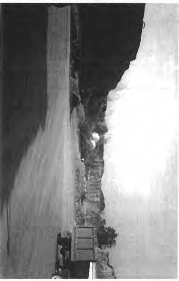
Retire to a safe distance. Each blast brings down c.20,000 tons of rock. 1958
