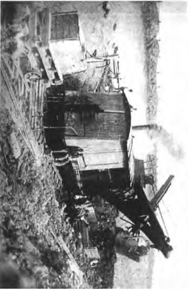
A steam navy at work on the Worthington to Ashby section of the Derby to Ashby railway. 1872
